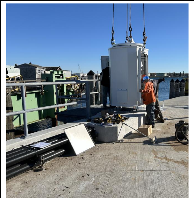
2754 - Setting Pedestal Base on Pier Foundation
