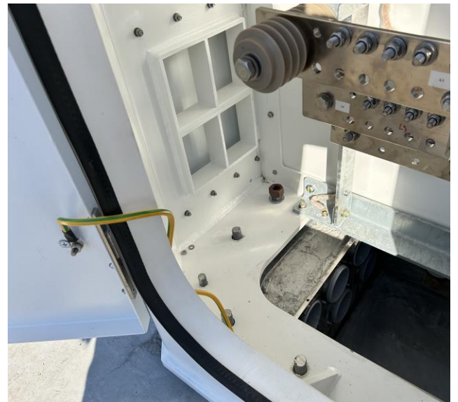
2762 - Aligning Bolts with holes in Pedestal
