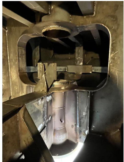
5174 - Rudder Post Area in Lazarette
