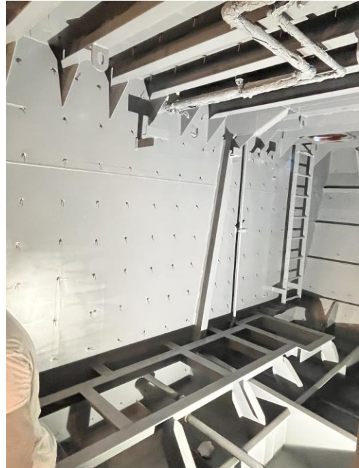
5238 – Switchboard Room Foundation Framing
