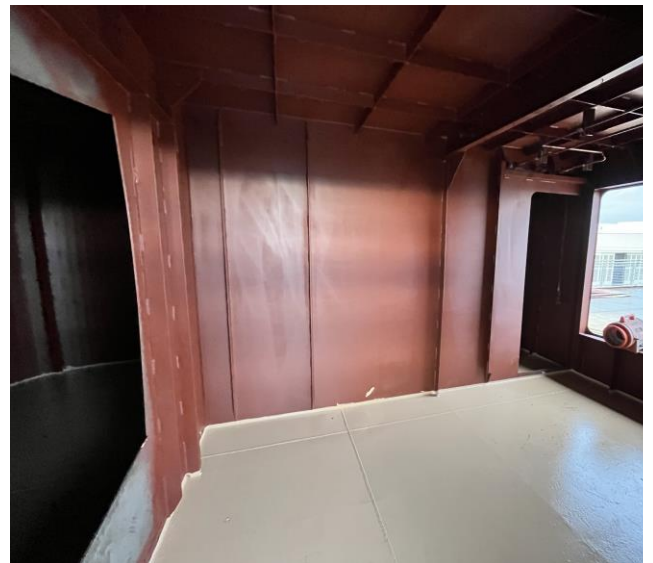
5160 – Paint Applied in Crew Locker Room
