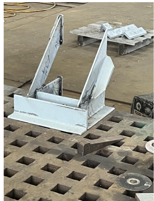
5185 - Equipment Foundation Framing being Assembled
