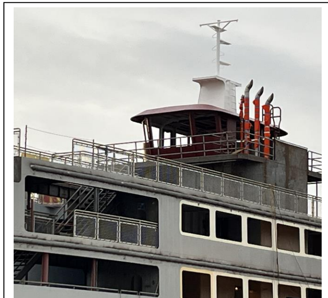
5151 – Starboard Side with Guards Installed and Windows Prepared
