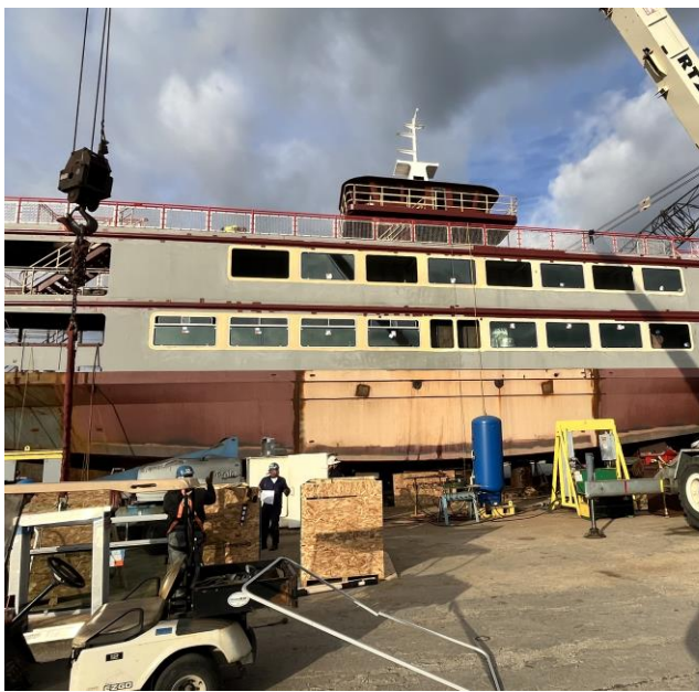
5306 – Some of the Operable Windows Installed in Port 01 Cabin
