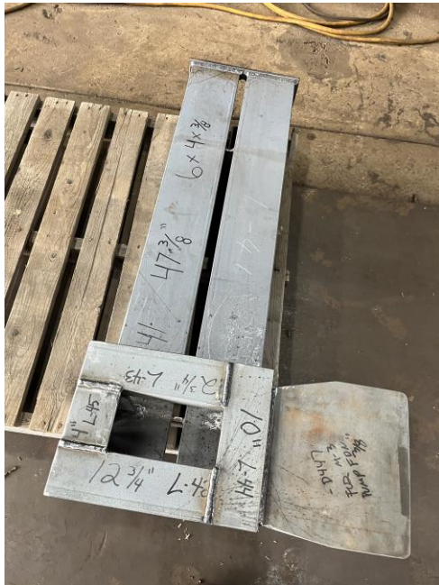
5179 – Equipment Foundation Framing being Assembled
