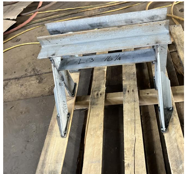
5182 - Equipment Foundation Framing being Assembled
