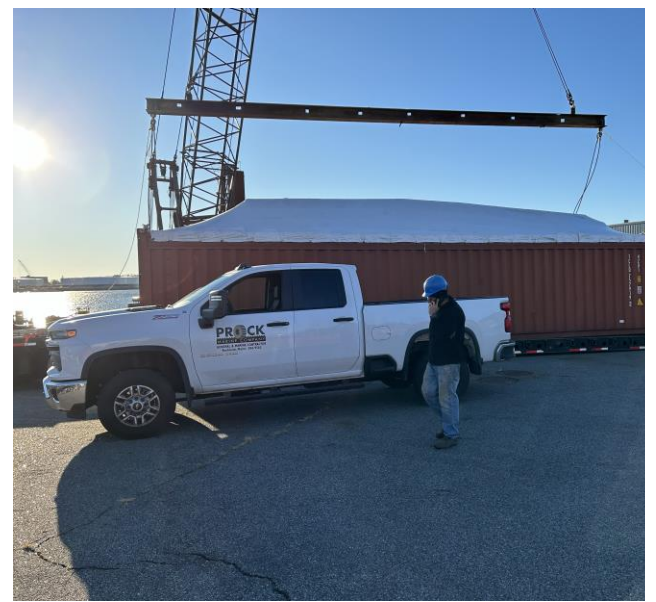
2731 – Preparing to Lift Container onto Barge
