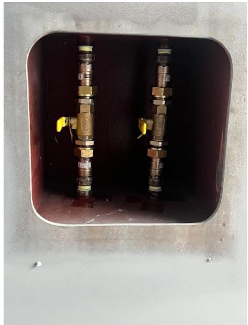
5132 - Installing Sprinkler Shutoff Valves
