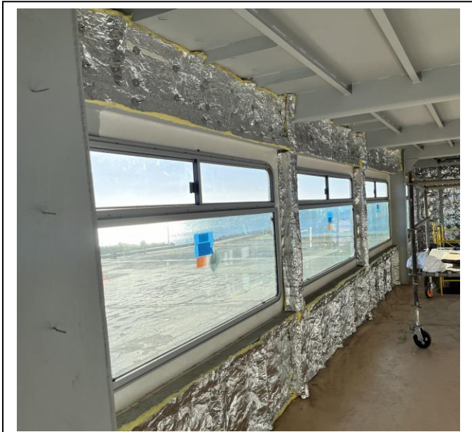
5341 – Insulating a Port Cabin after Window Installation
