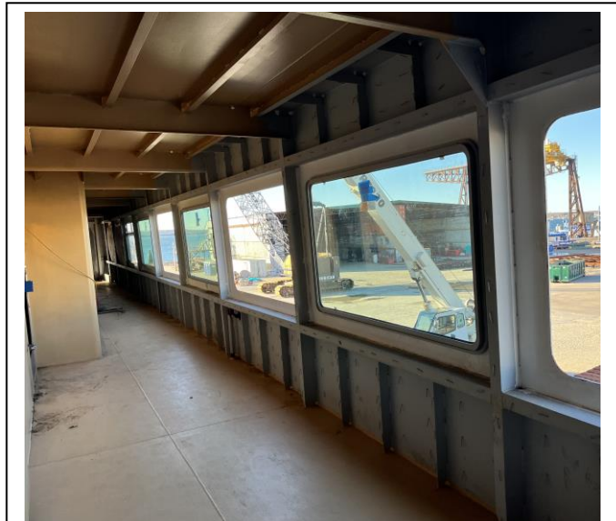
5344 – Windows Installed on Main Deck Starboard Cabin
