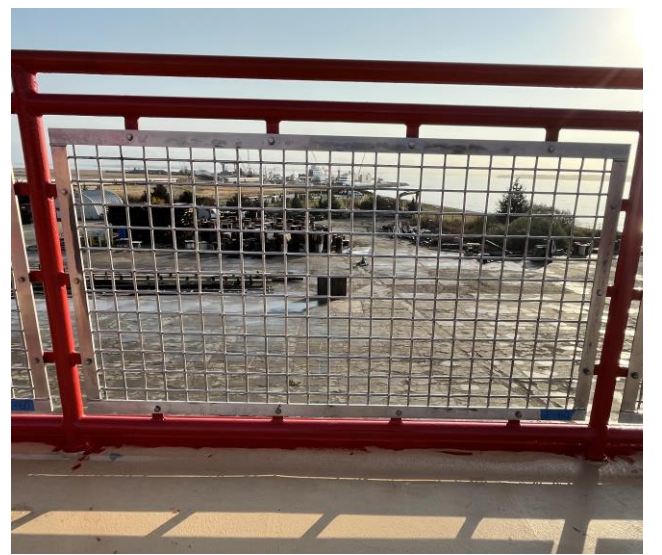
5271 - Handrails Installed on 02 Deck with Screen Sections in.
