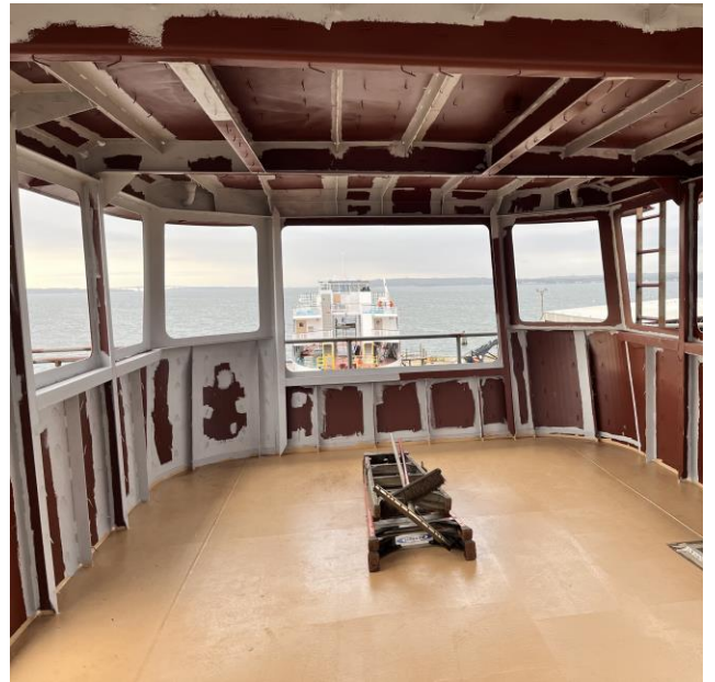
5162 – Painting Inside of Pilot House
