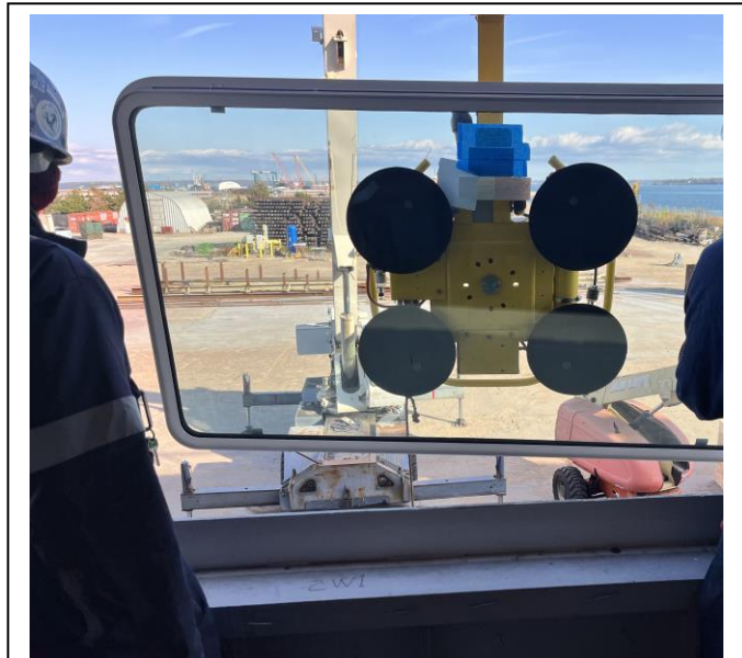
5256 - Installing a Widow
