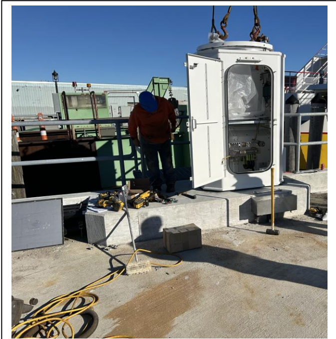
2759 - Setting Pedestal Base on Pier Foundation
