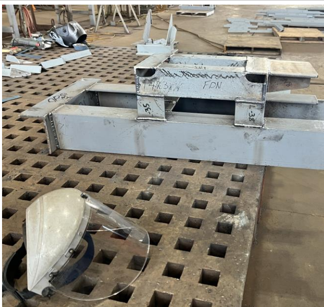
5183 - Equipment Foundation Framing being Assembled
