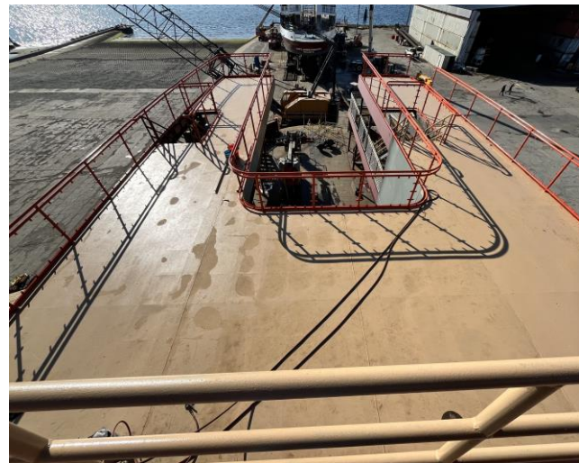
5242 - Painting a portion of 02 Deck
