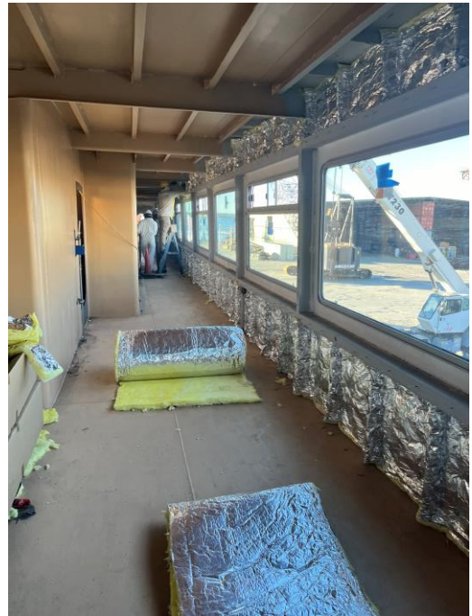
5357 – Insulating Starboard Main Deck Cabin
