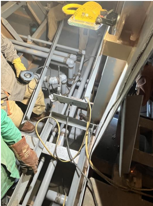
5237 – Installing Foundation Framing
