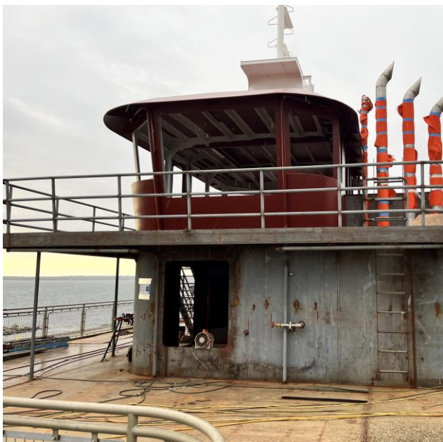
5159 – Starting to Paint Pilot House
