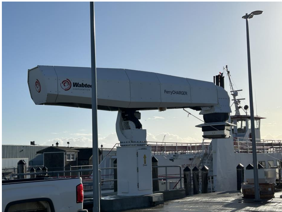
2795 – Charger in Place
