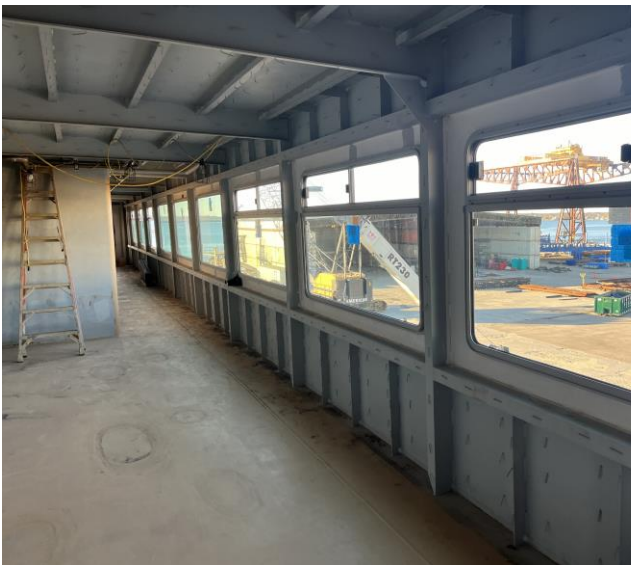
5358 – Windows Installed in Starboard 01 Deck Cabin
