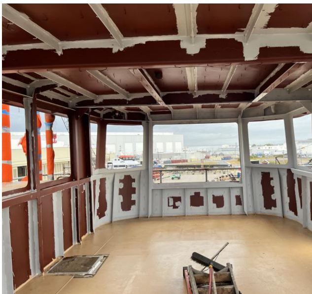
5163 - Painting Inside of Pilot House
