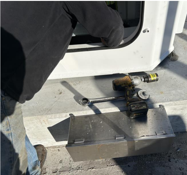
2761 – Aligning Bolts with holes in Pedestal
