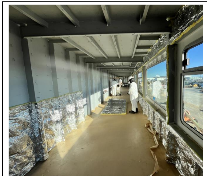
5343 - Insulating a Port Cabin after Window Installation
