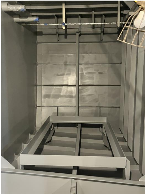
5155 - Paint Coating in Engine Room
