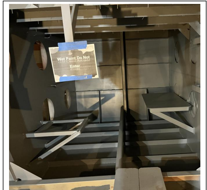
5152 – Paint Coating in Engine Room
