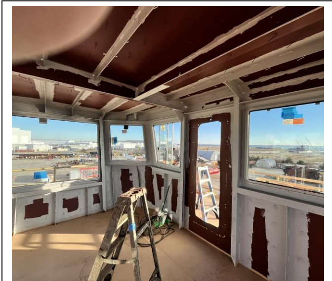
5374 - PH with Windows Installed
