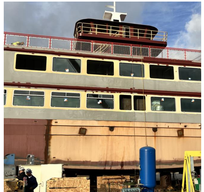
5307 - Some of the Operable Windows Installed in Port 01 Cabin
