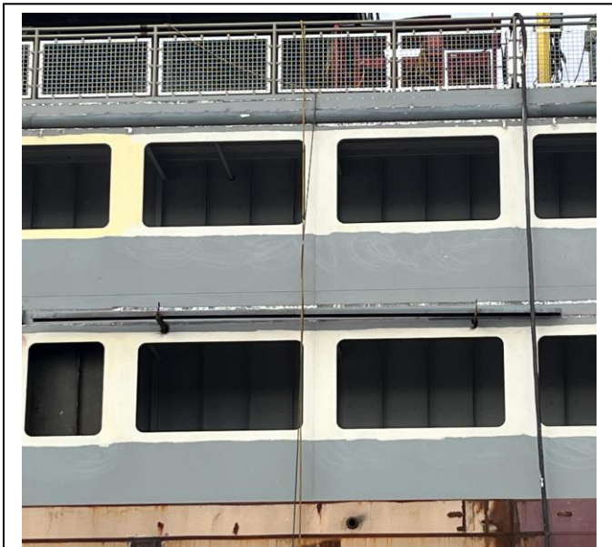
5142 – Window Openings being Prepared for Windows
