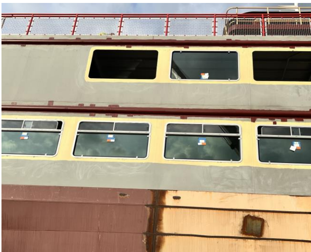
5308 - Some of the Operable Windows Installed in Port 01 Cabin
