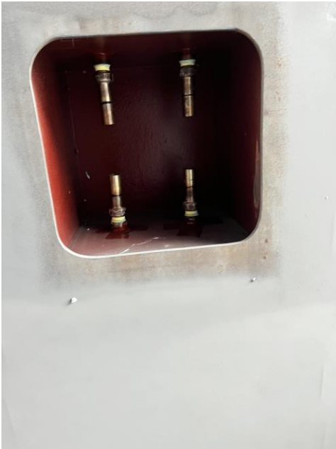
5123 – Installing Sprinkler Shutoff Valves
